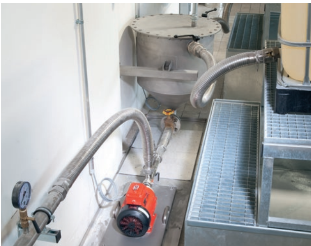
F 550 TR in action in the industrial sector – pumping viscous softener.
